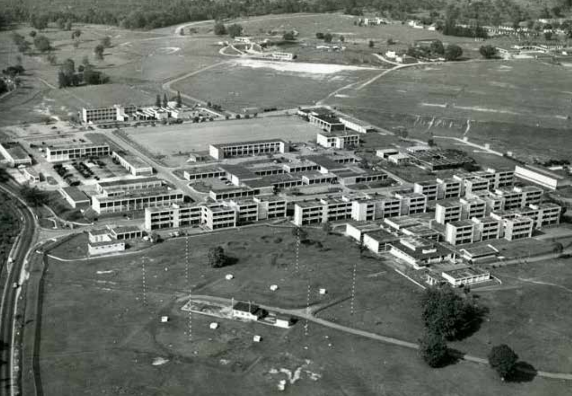
Aerial view of Dieppe Barracks
