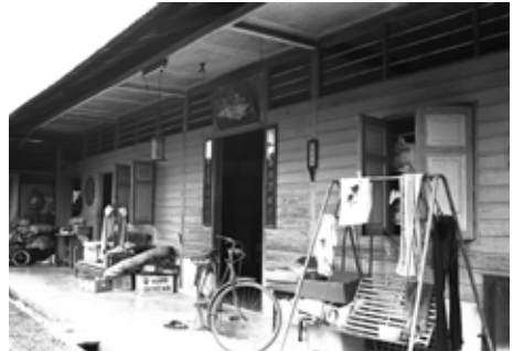
House in Kampong Amoy Kwee, 1967.
