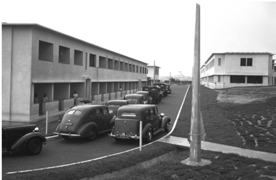
The newly built quarters for the Admiralty Asian staff at Singapore Naval Base, 1950.
